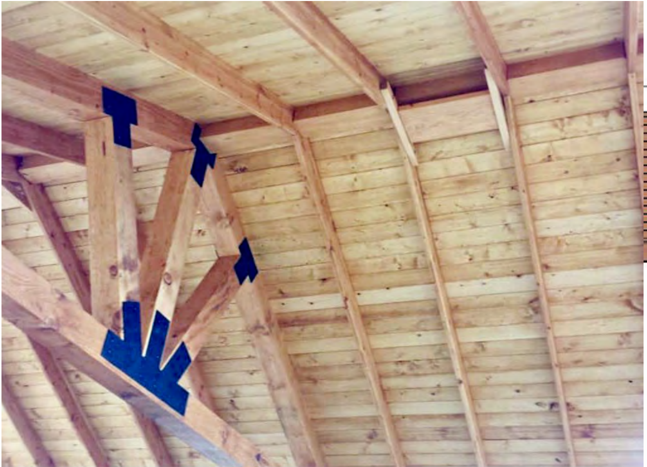
The Thick Timber Toledo Wood Pavilion (Options: 27' L x 25' W, Douglas-fir, 6-Post Anchor Kit for Gale-Wind, Electrical Wiring Trim for 2 Posts, 8 x 8 Supports and Posts, 8 x 8 Rafters, 2 Fan Bases, Transparent Premium Sealant). Photo Courtesy of T. Lane of Kingsburg, CA.
