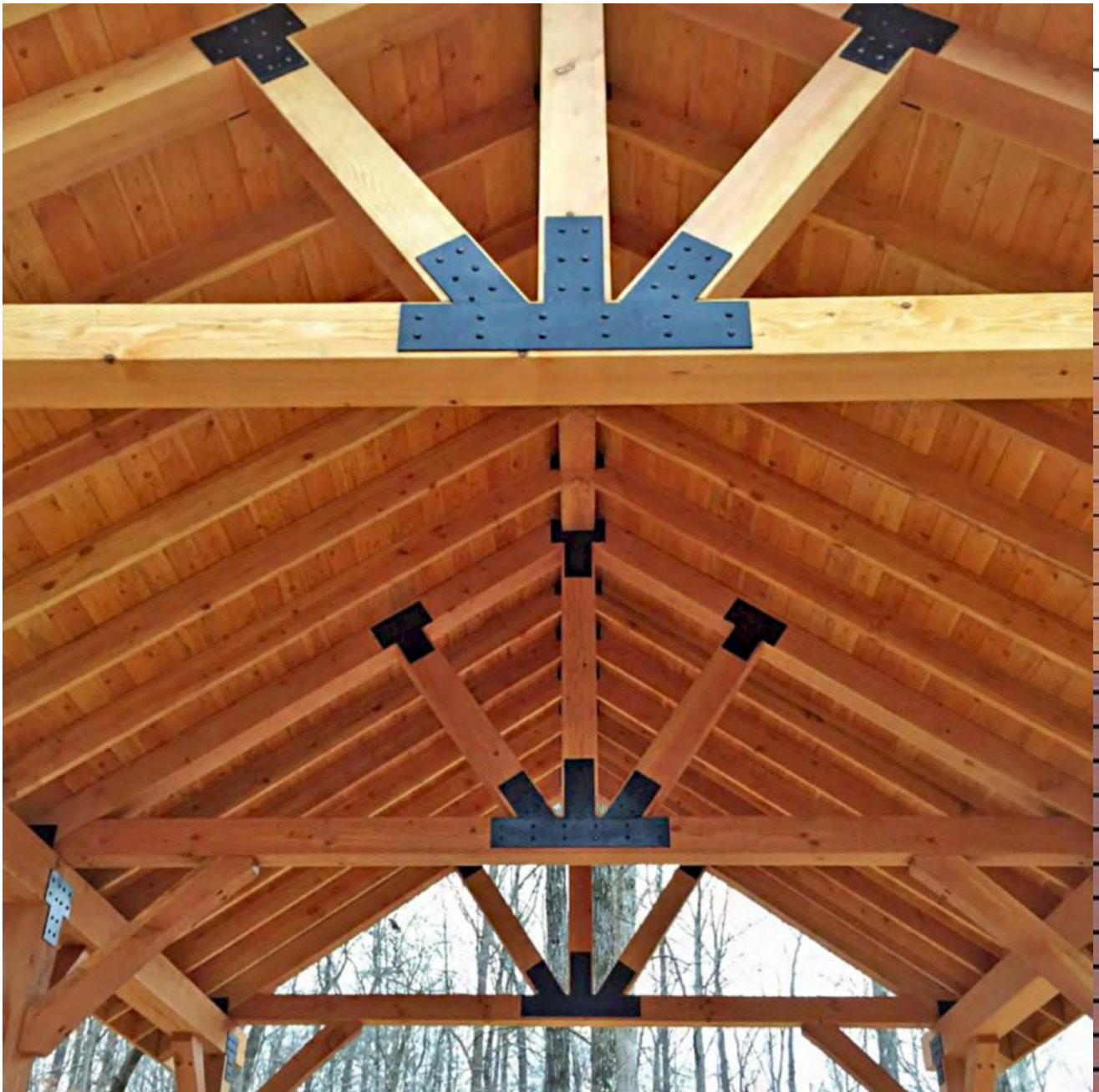
The Thick Timber Toledo Wood Pavilions (Options: 26' L x 20' W, Douglas fir, 6 Post Anchor Kit for Gale Wind, Electrical Wiring Trim for 3 Posts, 10 x 10 Supports and Posts, 8 x 8 Rafters, Transparent Premium Sealant). Photo Courtesy of M. Turner of Thaxton, MS.
