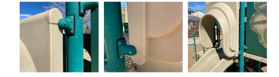
Issue IdentifiedThere is an entanglement or head entrapment hazardRecommendationAddress the issues immediately. [ASTMI 1487] View ASTM Site
