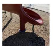
Positive Finding Issue Identified Recommendation Loose-fill surfacing materials have no foreign objects or debris Loose-fill surfacing materials were displaced under heavy use areas Replace the surfacing material. [reference ASTMI 1487, CPSC] <u>View ASTM Site</u> **Notes:** There is a lot of displacement of surface material. Someone should come out at least weekly to make sure surface material has not been displaced.
