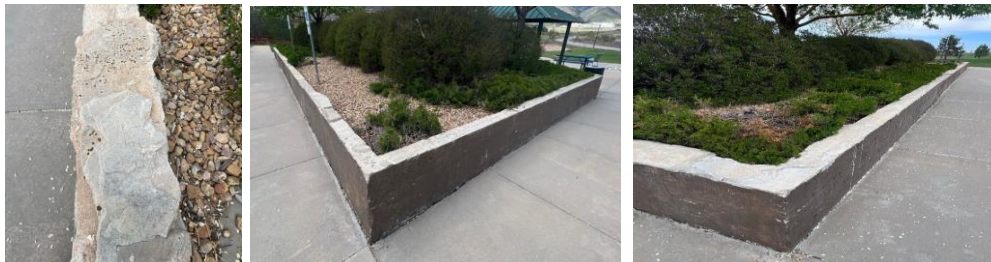
Existing Conditions Of Planter Wall
