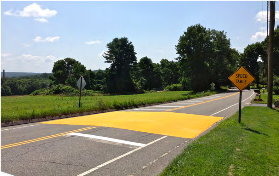
Example of traffic calming element
