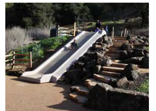
11 CONCRETE EMBANKMENT SLIDE (age varies depending on slope)
