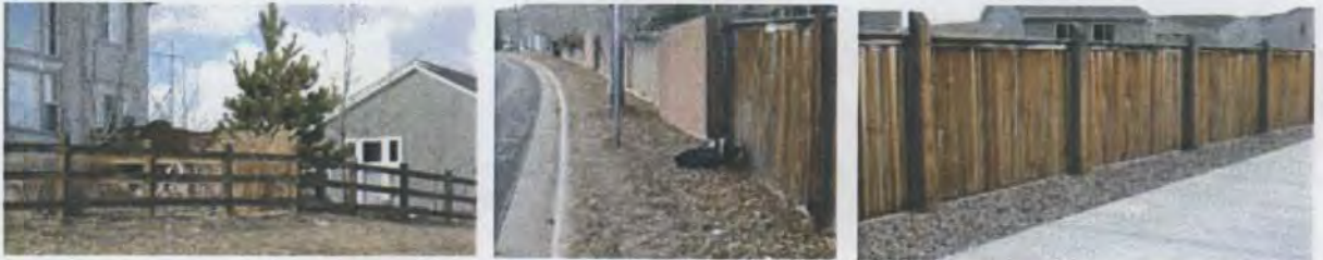
There are multiple types of fencing along Village Circle West
